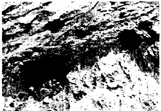
Fig. 7. Potholes on a shore platform in Seogeon-do.
