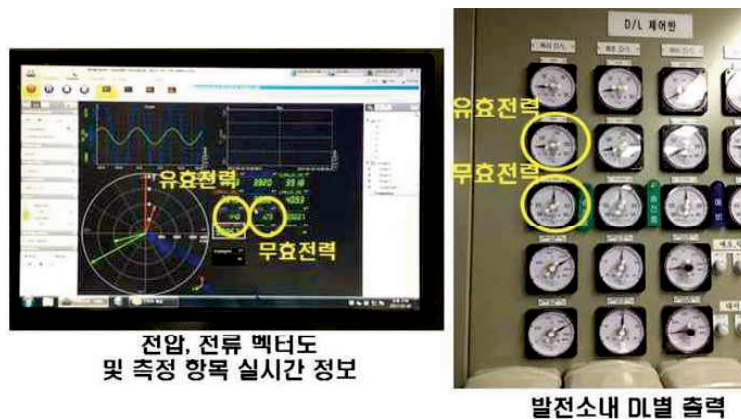
Fig. 7 Comparison between power quality analyzer output and power plant output
