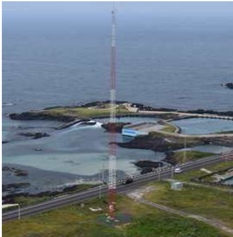
Fig. II-8 80 m tall met mast in Haengwon wind farm
