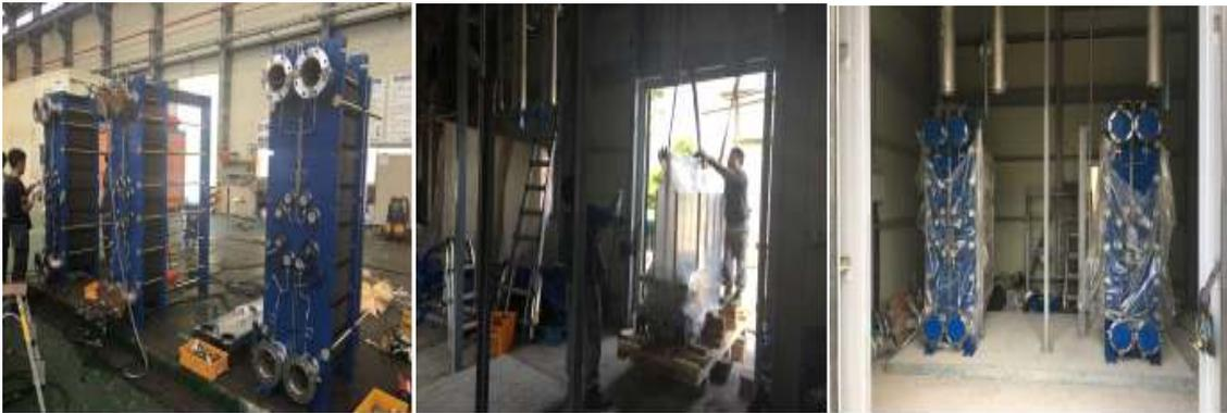
Fig. 5 Plate heat exchanger installation
