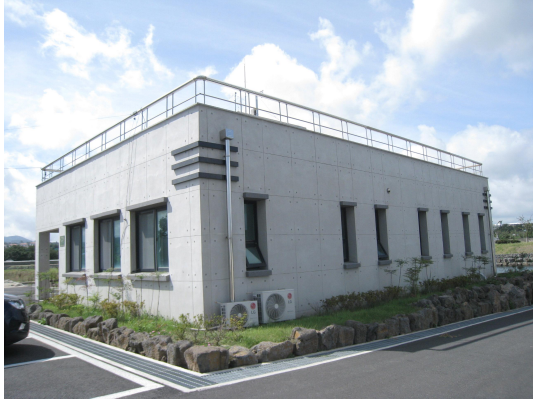
(a) pumping station building
