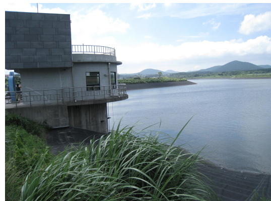
(b) intake tower
