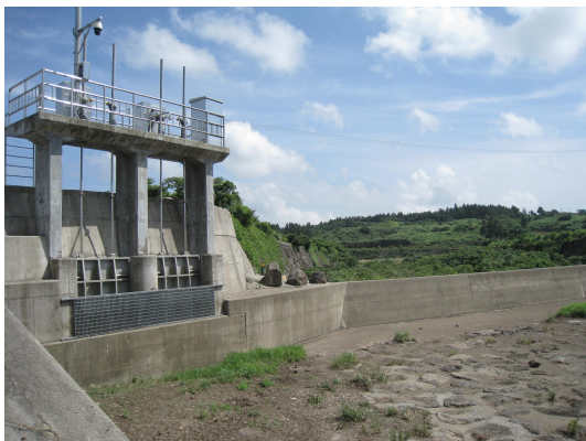
(a) intake gate and diversion weir
