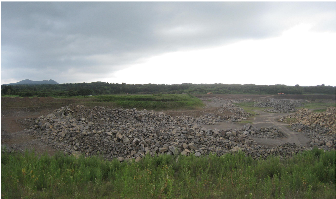
Fig. 3.25 Hamdeok reservoir during excavation
