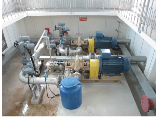
(b) pump installation
