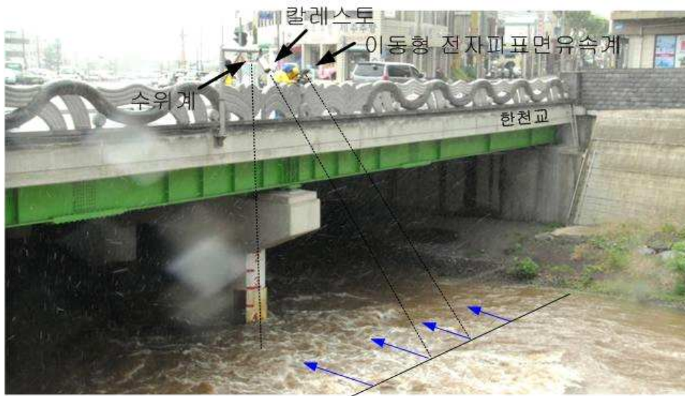
Fig. 4.2 Observation of stream runoff using observation equipment
