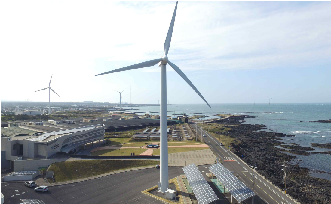
Fig. 1 Fixed rotor speed type wind turbine(Vestas V47)
