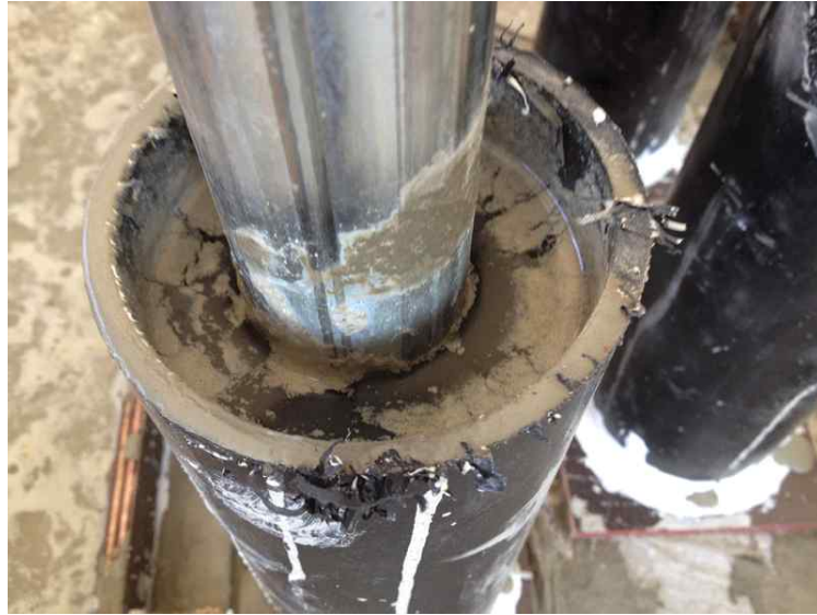
Fig. 5.5 Bleeding of grouting material
