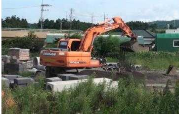
Fig. 3.7 Excavator work to bucket
