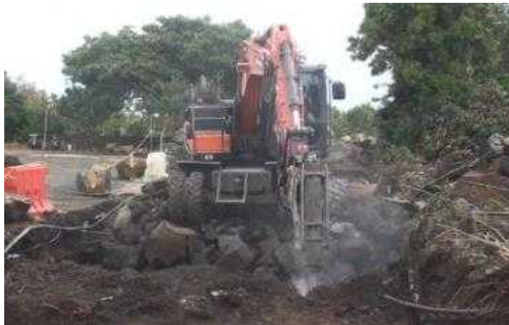
Fig. 3.8 Excavator work to breaker
