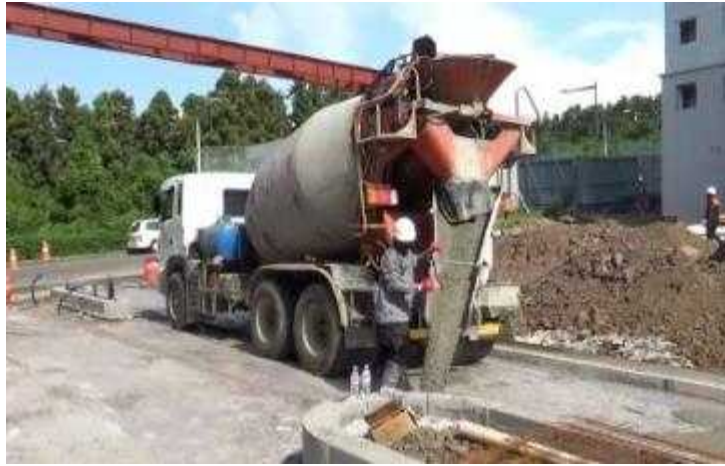
Fig. 3.9 Concrete mixer truck to work
