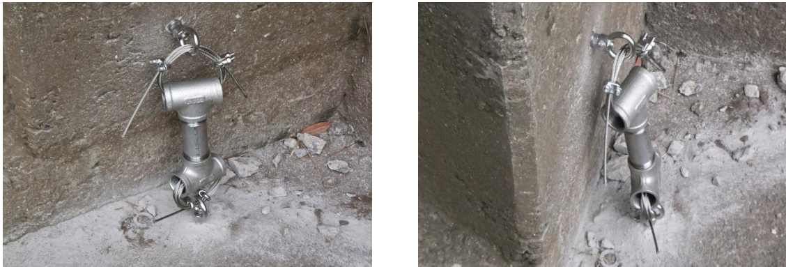
Fig. III-13. The position of DIVER-water gauge
