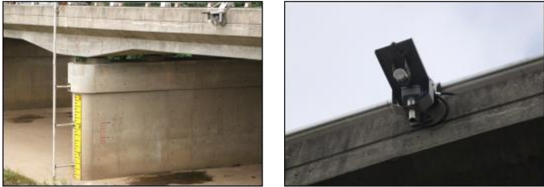
Fig. III-14. Kalesto installed at Seong-eup bridge
