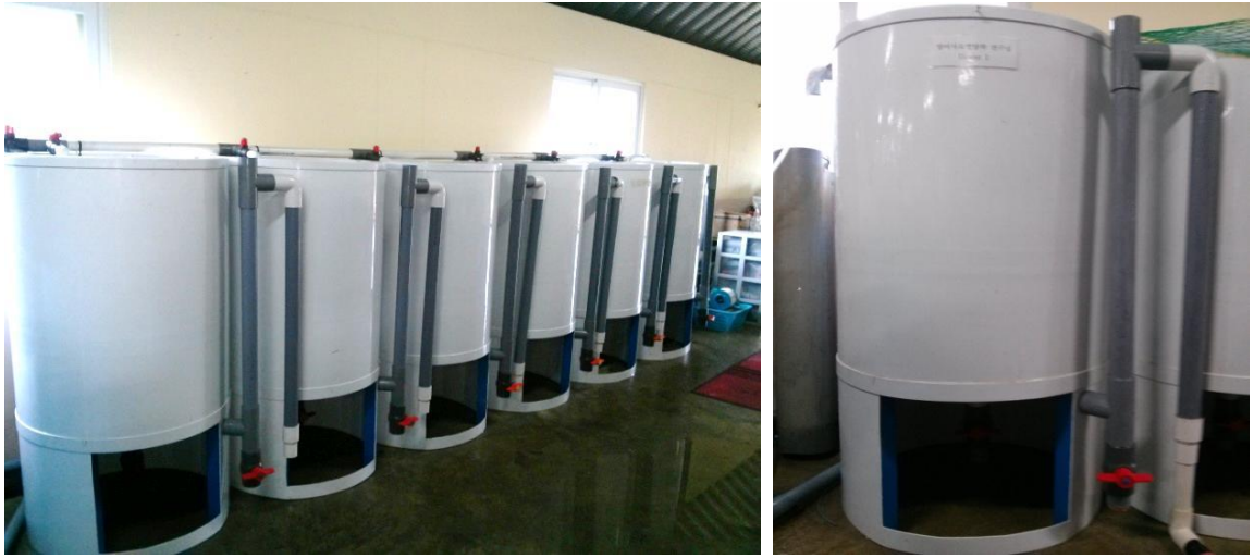
Figure 1-3. Feces collection tanks (Guelph system)
