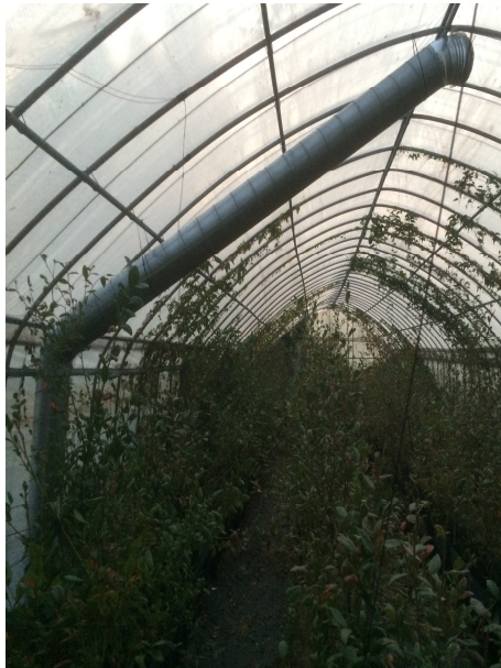
(a) Suction duct for surplus heat of the green house
