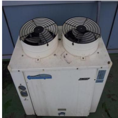
(b) 3HP class condensing unit
