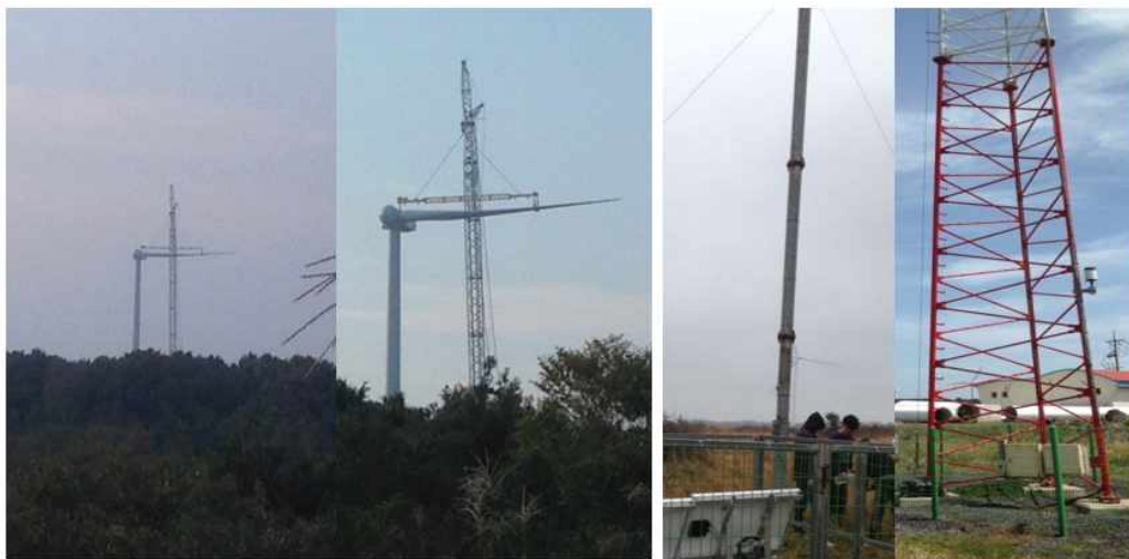
Figure 1-2 Assembling of 80m hub height wind turbine (Left) and Tubular and Lattice type Met-Masts (Right)
