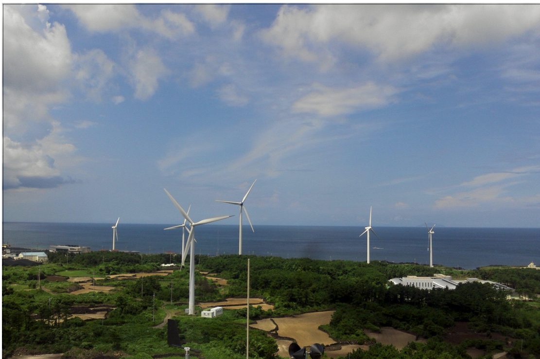
Fig. 7. View of A wind farm close to the sea (Total capacity of 11,450kW)
