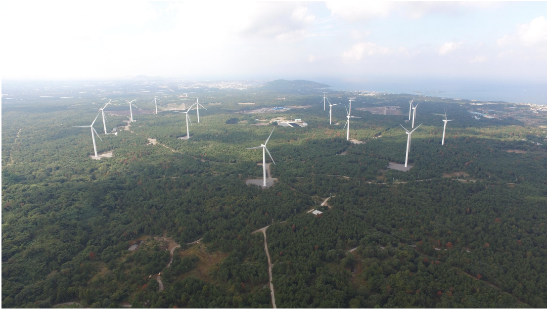
Fig 10. View of D onshore wind farm (Total capacity of 30,000kW)
