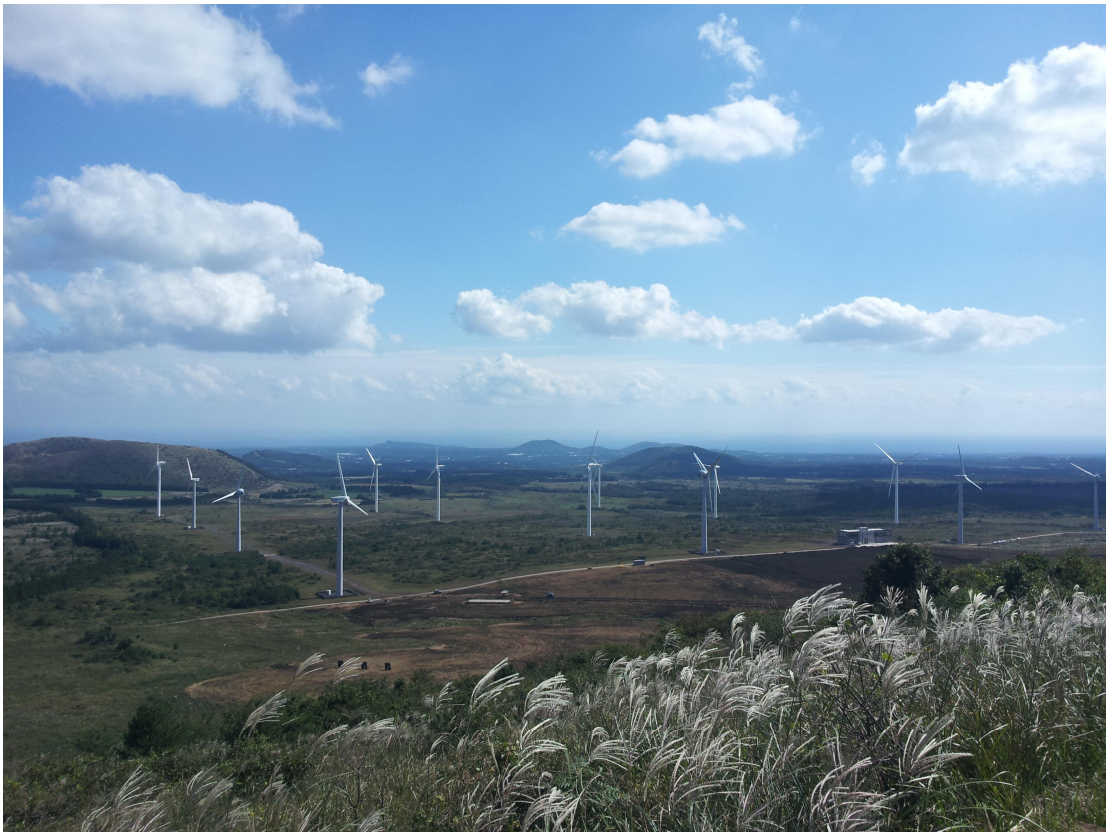
Fig 11. View of E onshore wind farm (Total capacity of 15,000kW)
