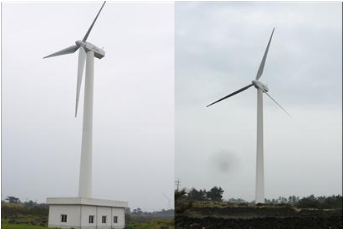
Fig. 9. View of C wind farm near the sea (Total capacity of 1,700kW)
