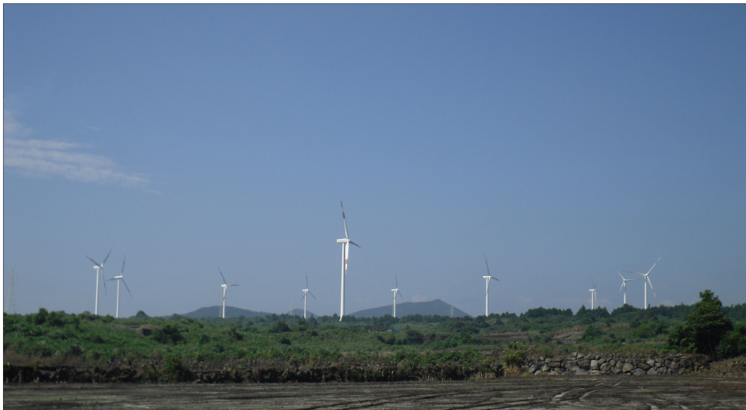
Fig. 3.1 View of Sung-san wind farm
