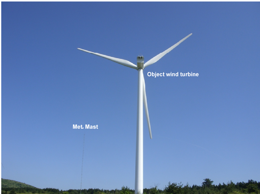
Fig. 3.26 Met. Mast and wind turbine for measurement of velocity deficit and turbulence intensity in a wake
