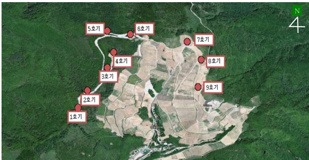
Fig. 3 Layout of wind turbines in Taebaek wind farm
