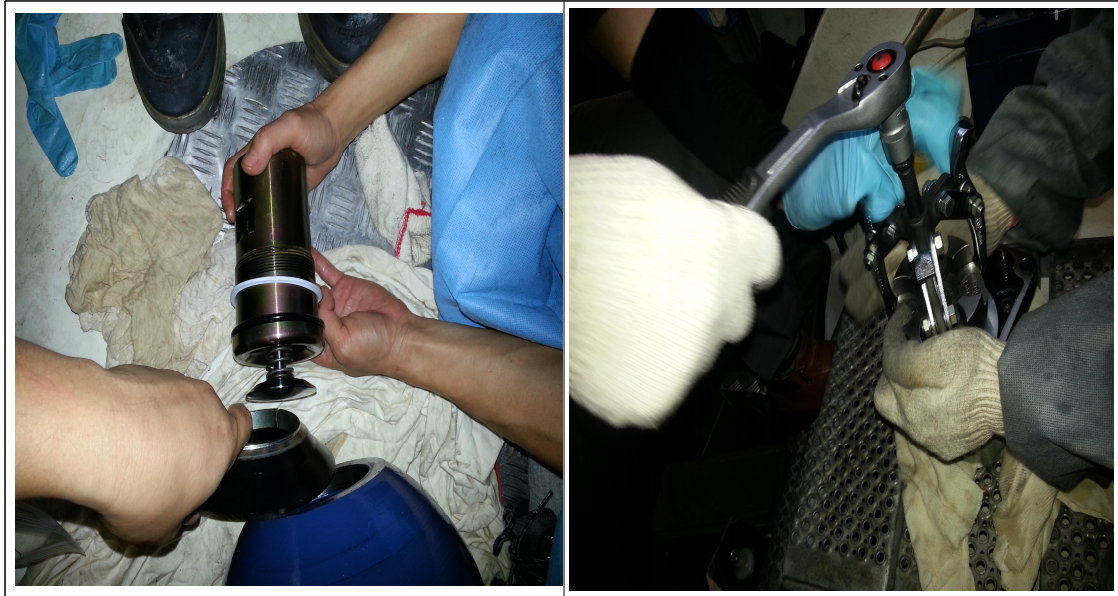
Fig. 20 Bladder & hydraulic pump repair No. 4 & 6 wind turbine at Sungsan wind farm
