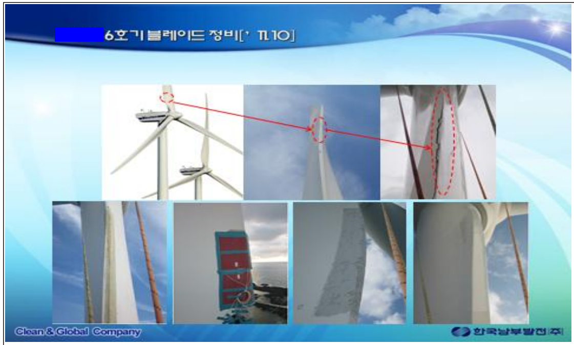
Fig. 18 Blade repair of No.6 wind turbine at Sungsan wind farm
