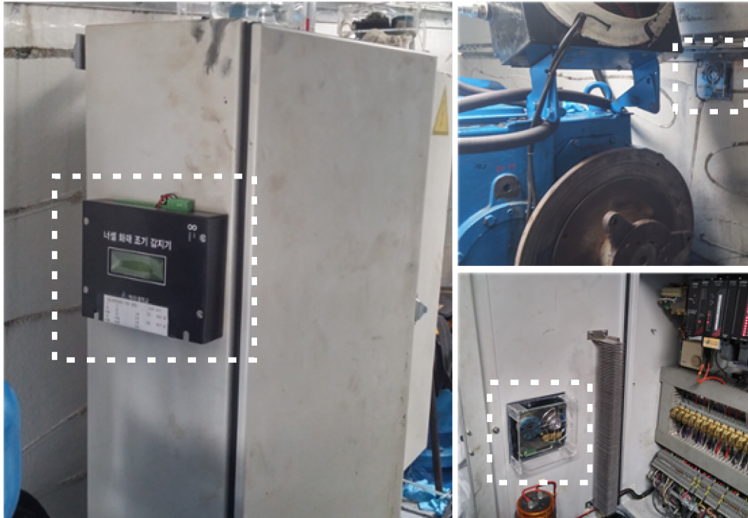
Fig. 36 Fire detection system installation
