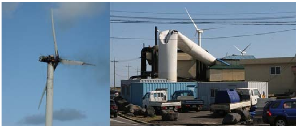
Fig. 2 Jeju wind turbine fire
