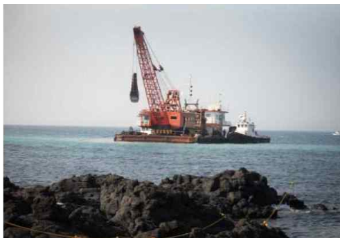
Fig 12. The trenching method of Woljeong offshore wind.
