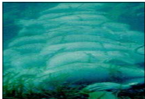
Fig 26. Concrete bag. [16]
