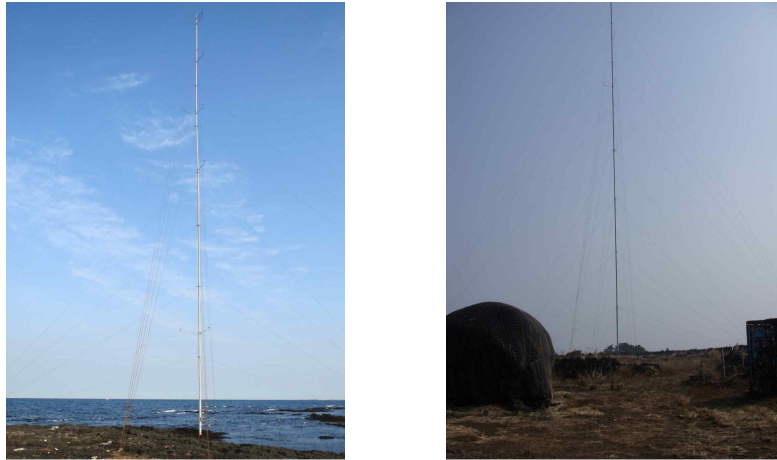
Figure 3.11 Met-mast (left: Handong, right: Pyungdae).
