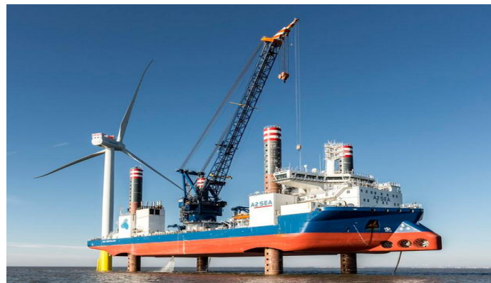
Figure 16 Jack-up vessel Sea Installer [28].
