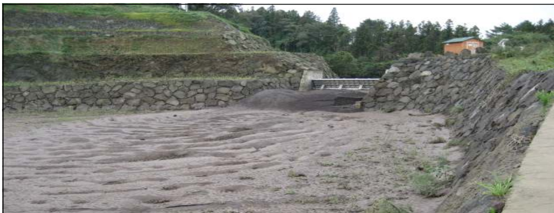
Fig. 11. The front sediment view of the inlet of the HanCheon1 Retention pond in HanCheon.
