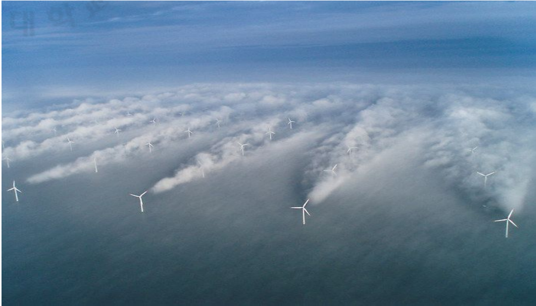
Fig. 1 Illustration of wake at offshore wind farm in Horns Rev in Denmark[8]
