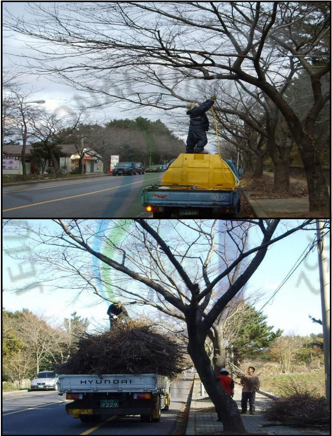
Photo 6. Sterilization treatment and disposal of cut branches after the removal work completed.
