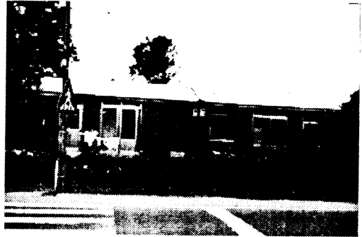
Fig. 6 An outside view of Urban Type House for The sufferers (Located at Bong-gae, 1959)
