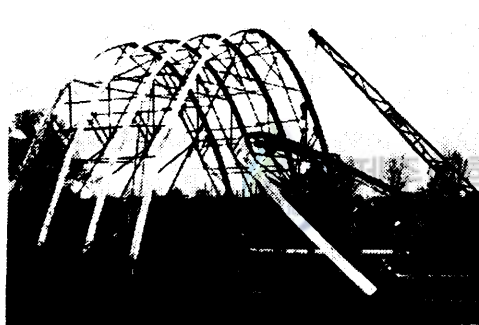
Fig. 36 A building process of the Sam-an type house
