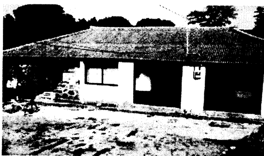
Fig. 53 A outside view of house reconstructed
