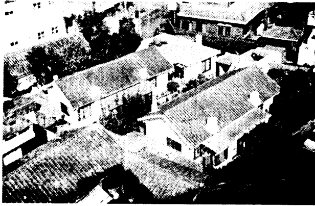
Fig. 14 An outside view of Welfare House (Located at Samdo-Idong)
