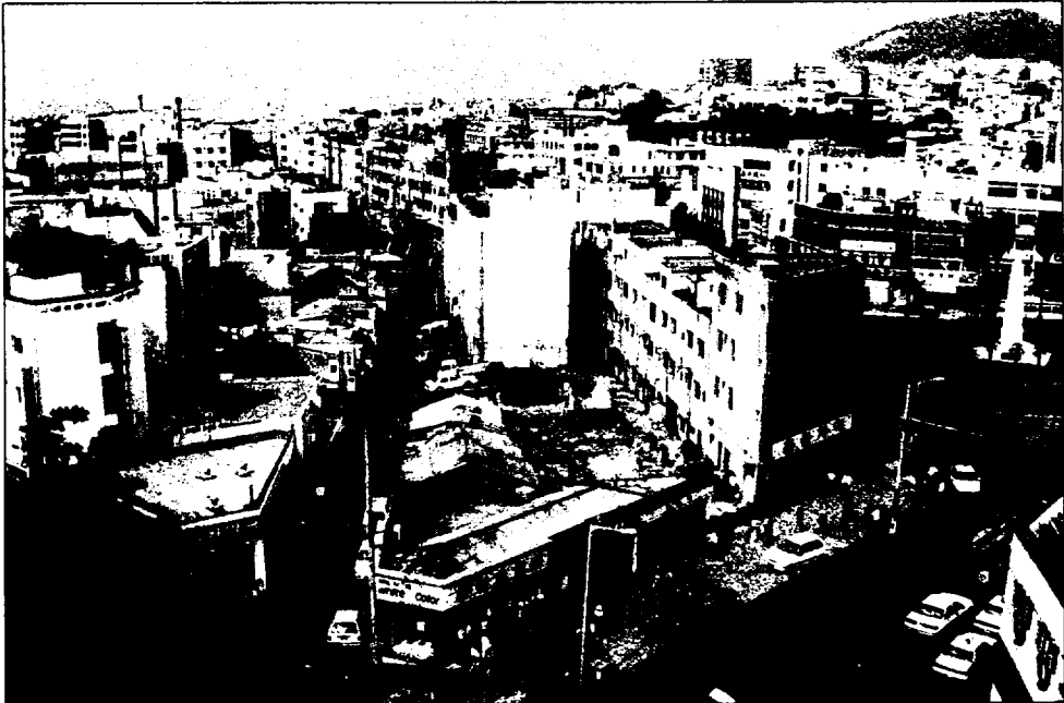
Fig. 8. Sanji stream before demolition
