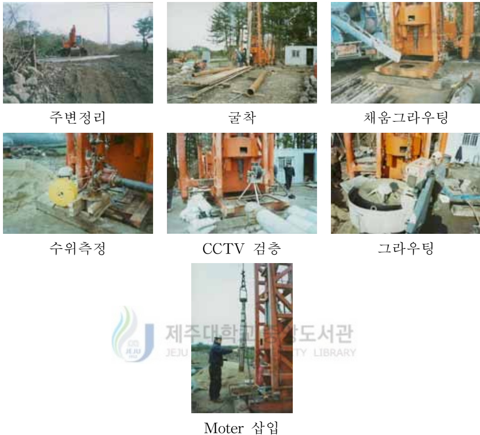
Fig. 12. Feature of operations in Seogimnyeong #2 District
