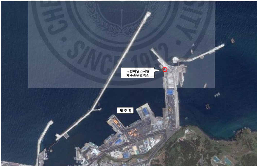
Fig. 2 Location of Jeju Tidal Station(Google Earth, 2007)
