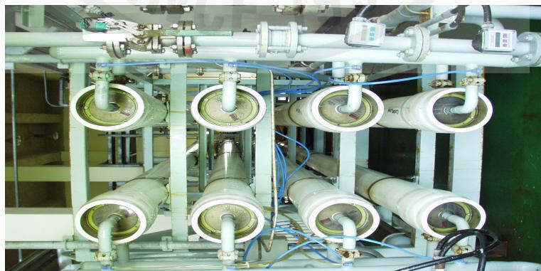
Fig. 13. RO Device installed in Water Conversion Facility in Udo Island(제주도, 2003)
