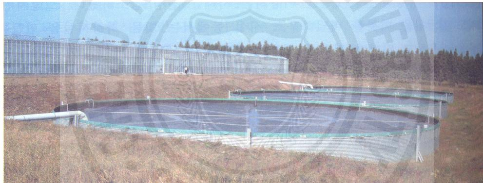
Fig. 26. Rainwater Storage Facility of Glass Greenhouse in Korea Airport Service, Co.
