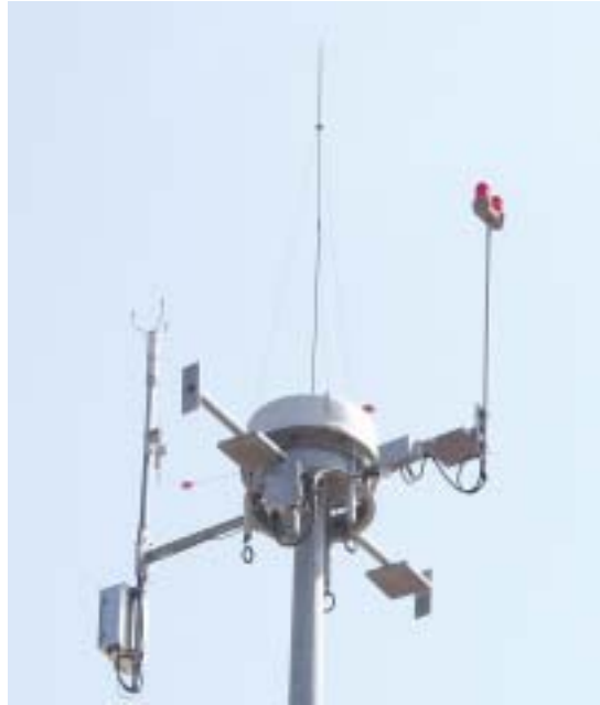
Fig. 12. LLWAS remote station
