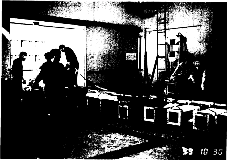
Photo 4 Compact of concrete.
