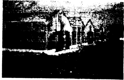
Fig. 4 An outer appearance of plastic greenhouse
