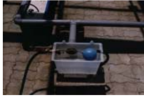
Photo 2. The connected state of nutrient supplying tube. (Φ50mm PVC tube)
