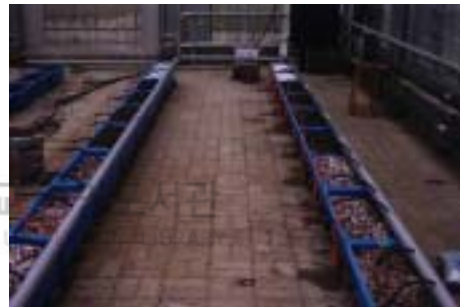
Photo 4. The installation scene of capillary supplying system.
