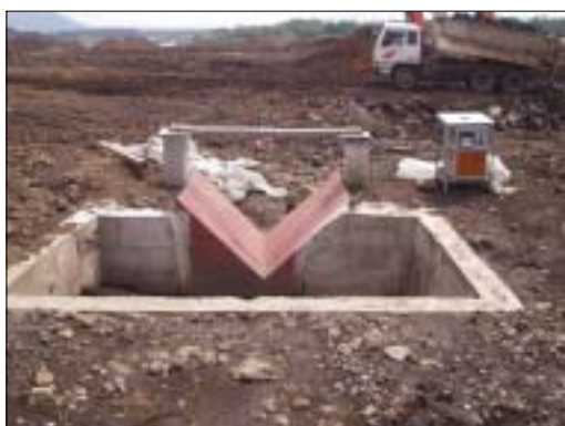
Fig 4.1 Setup of water level gauge
