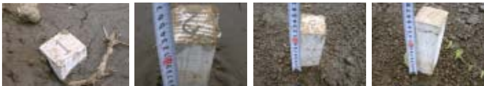
Fig 4.13 Piles after rainfall in II·III zone
