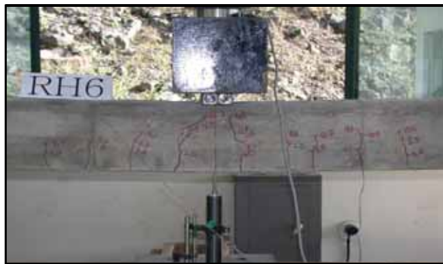
Fig. 6.13 Crack pattern of RH6 experimental specimen
