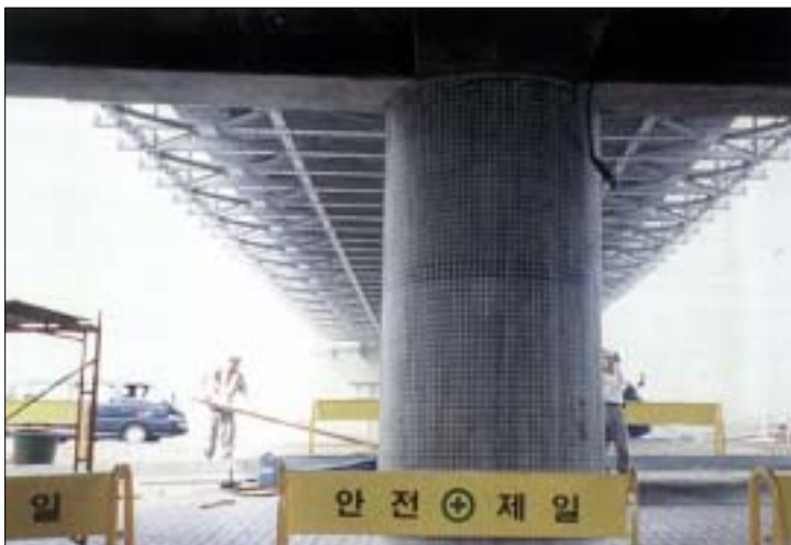
Fig. 2.6 Application of NEFMAC method using CFRP grid
