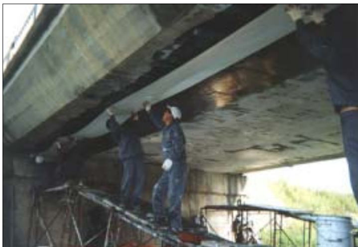
Fig. 2.3 Application of external bonding method using CFRP sheet
