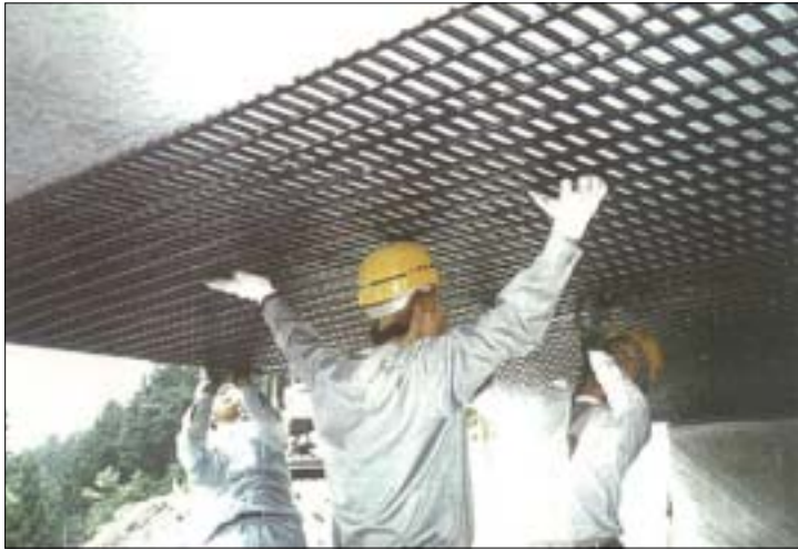
Fig. 2.5 Application of NEFMAC method using CFRP grid
