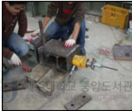
Fig 4.8 Jacking view of tendon
