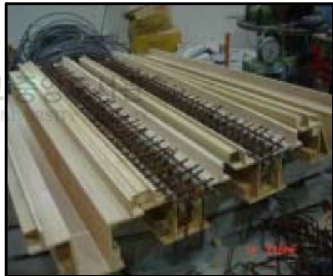
Fig 4.6 Fixing steel as form
