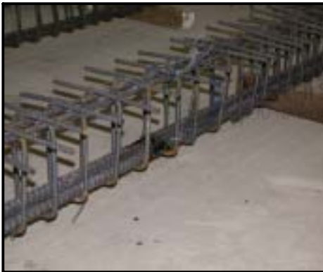
Fig 4.5 Arrangement for stirrups
