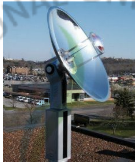
Figure 9: General view of the Hybrid Solar Lighting System
