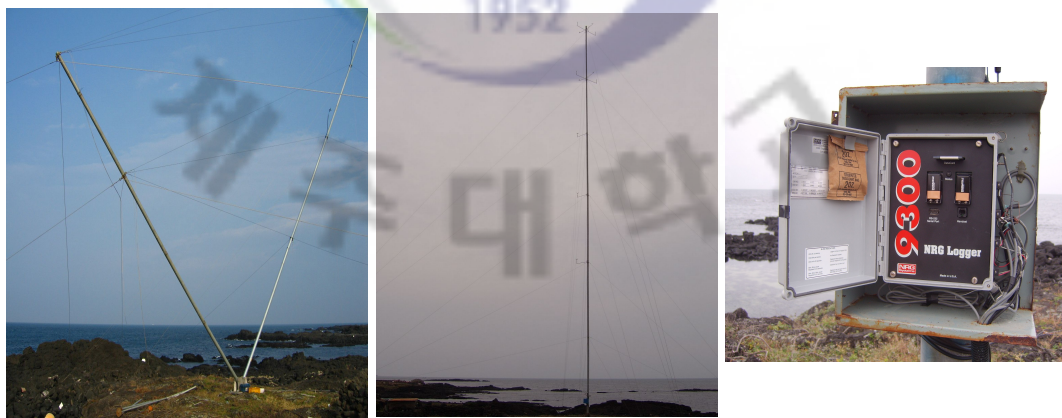
Figure 3.11 Mast installation and logger type
